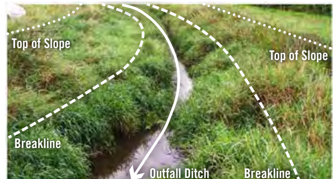
Figure 10.2 Outfall Ditch Survey Example Less Than 3ft
