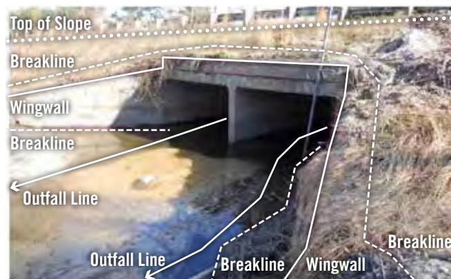
Figure 10.7 Culvert Survey Example
